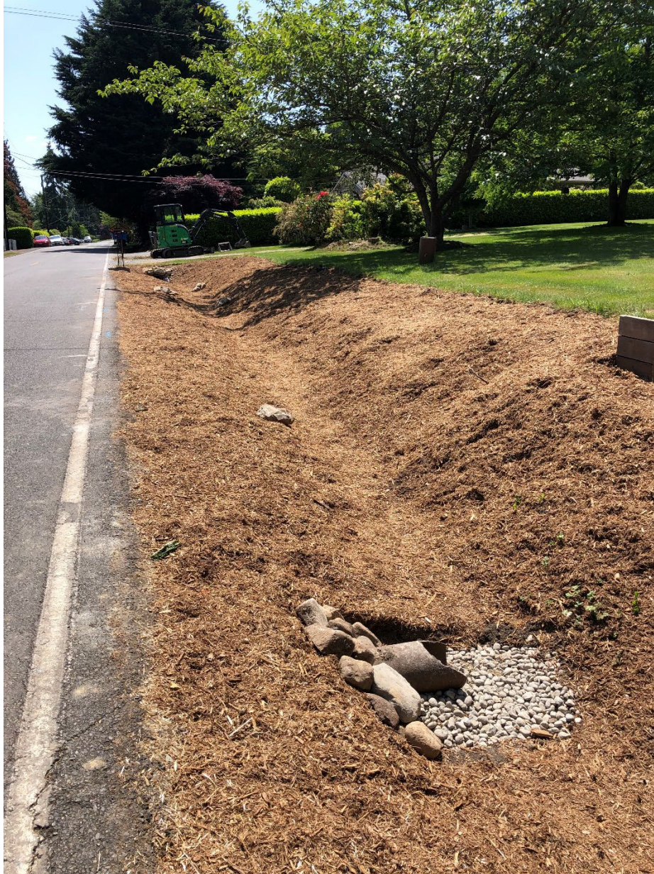
This bioswale will significantly reduce (or eliminate) the stormwater runoff from 83 rd Avenue from directly flowing into the Perrinville Creek watershed. [Photo taken June 1, 2023]
